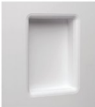
Alcoves become easy to form accurately with Fiberock for all components. Bond the edges and the back of the alcove to the reverse face of the wall lining, and then rout (using the sides as guide) out the front lining to accurately form the desired corner profile.
